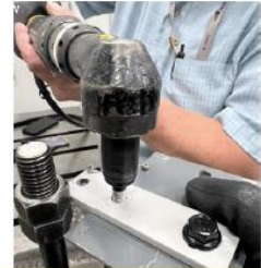
Pre-driven bolts (Torqued to 25 Nm into a steel nut and then backed out)
