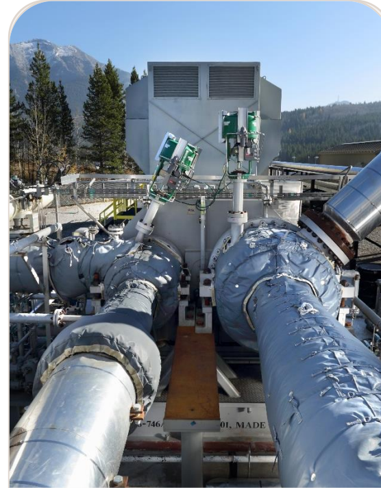
Two-stage Expander EEGI4/6 7.3MW, Butane, Canada, 2013
