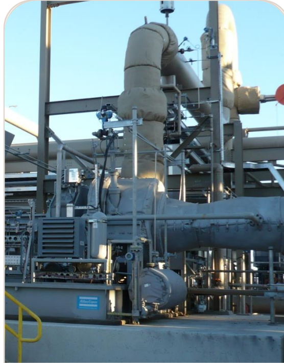
Single-stage Expander EGI8 15MW, i-Butane, USA, 2007
