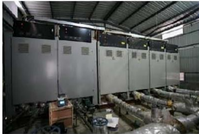
Factory Fabricated for Apartment Building, One Day Heat Storage, China, Electric Heat, Up to 8 MWh
