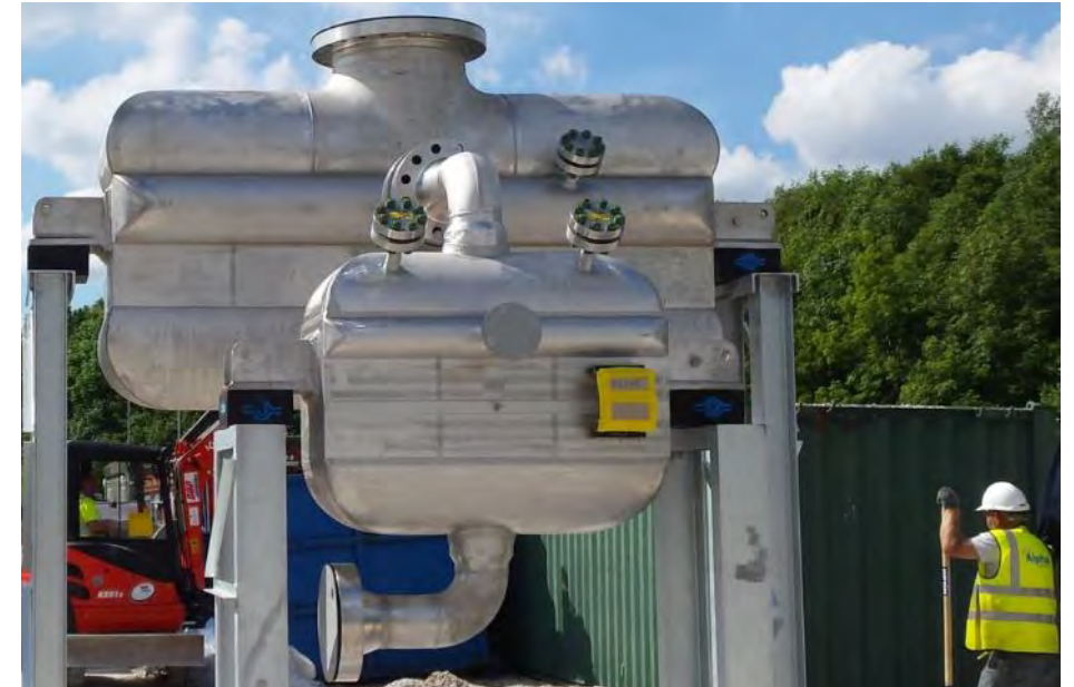
Bury Demo site Evaporator and HX1 (front)
