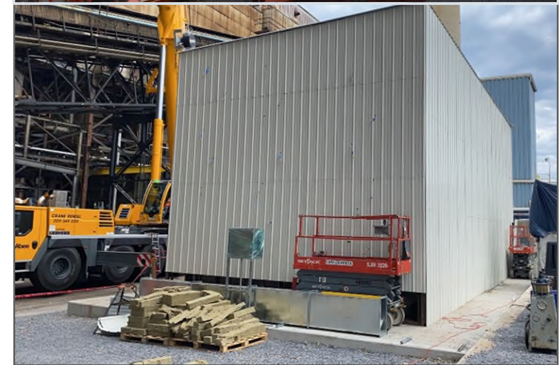
Gaston after installation of insulation and cladding
