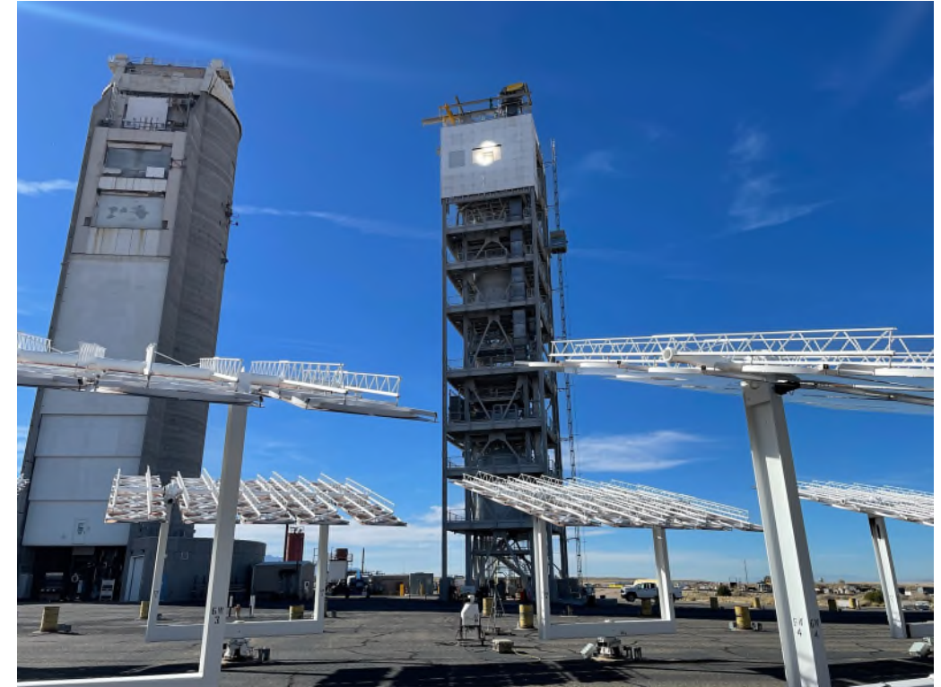
Sandia National Laboratories' Gen3 Particle Pilot Plant (G3P3) 775 °C flowing particles TES system. 6 MWh demonstration.
