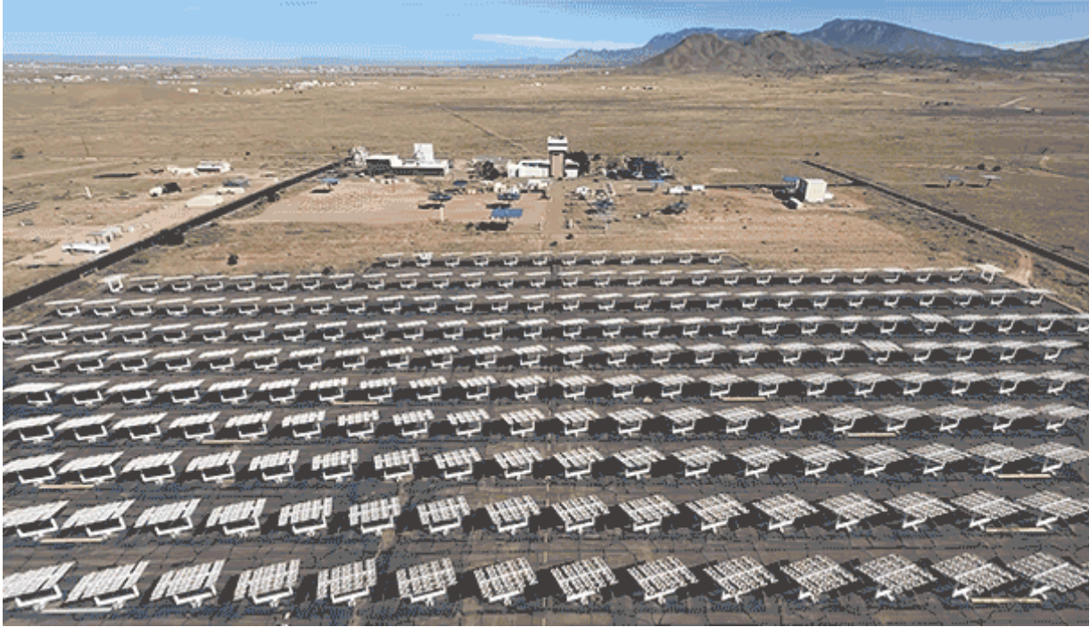
Sandia National Laboratories' Gen3 Particle Pilot Plant (G3P3) 775 °C flowing particles TES system. 6 MWh demonstration.
