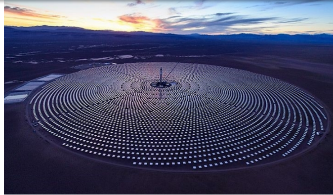
Solar Reserve's Crescent Dunes (100 MW e ) 1.1 GWh e Thermal Energy Storage
