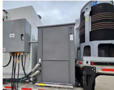
Power Distribution for easy site or generator connection and all chilling/HVAC on trailer
