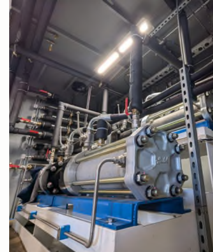
Compression on Trailer up to 700 bar
