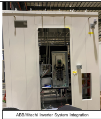
Fuel cell system (left) and inverter (right) integration at GPC
